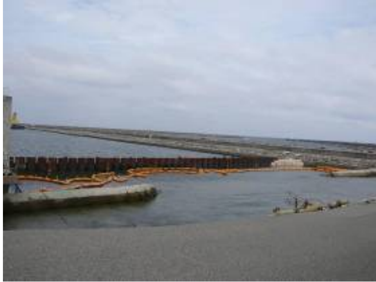
Status of steel pipe sheet pile
